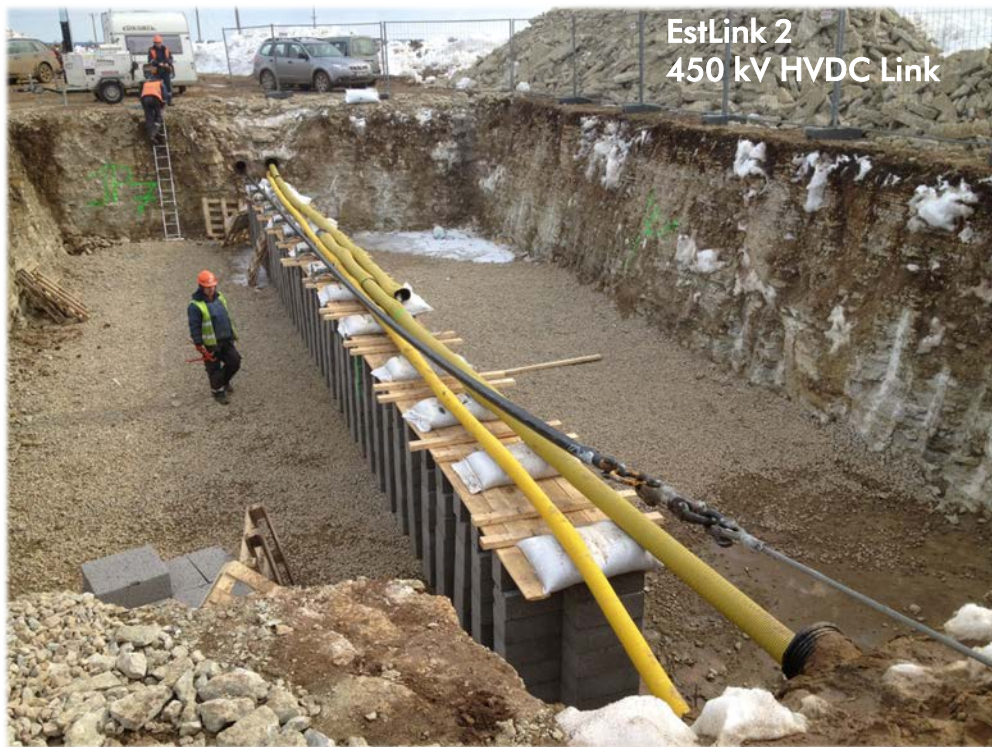
Cable pulled through a PE-pipe into the jointing pit
