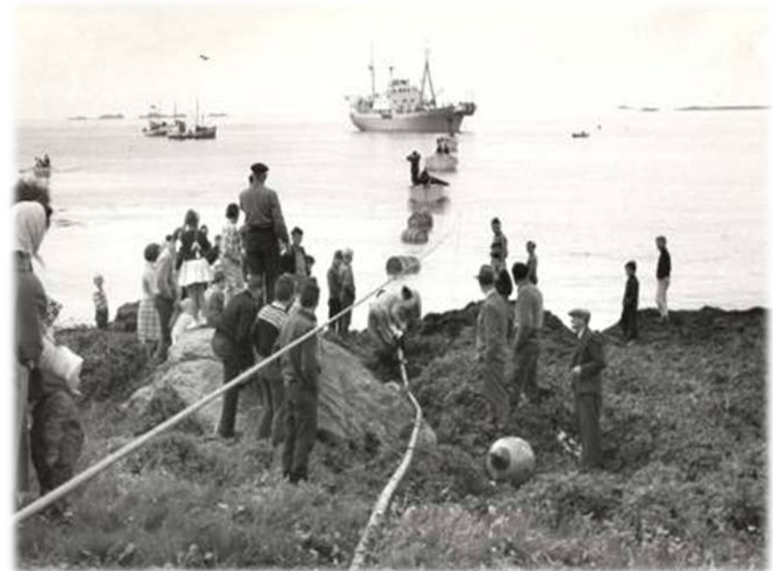
Submarine cable installation in the fifties
