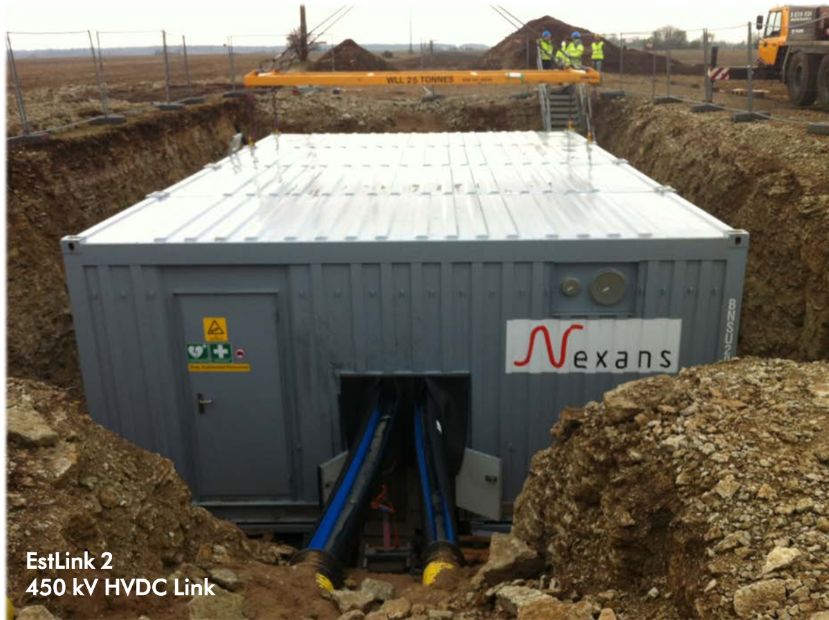
On-site preparations of the jointing pit
