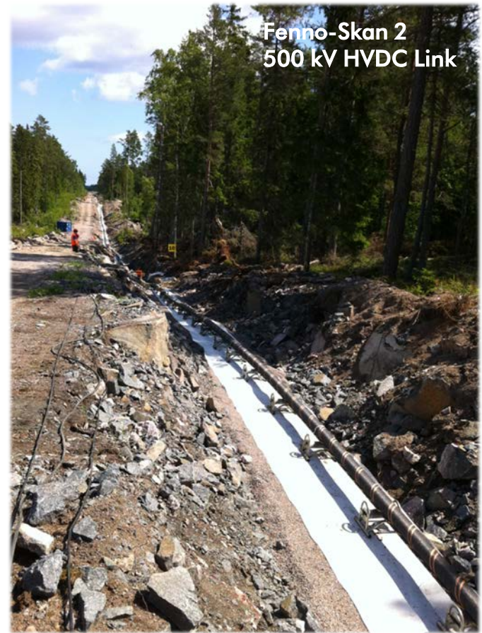
Cable pulled in an open land trench
