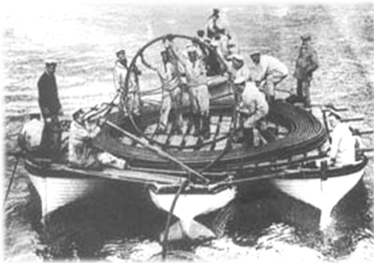
Submarine cable installation in the thirties
